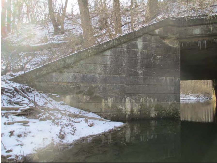
15: General View of the Near Right (Southeast) Wingwall
