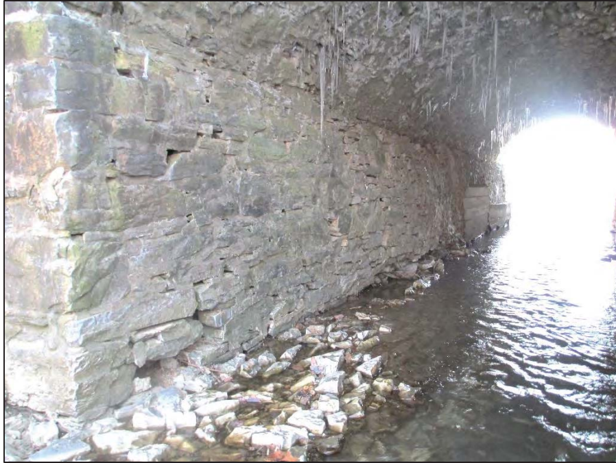
19: General View of the Far (North) Abutment, Looking Upstream
