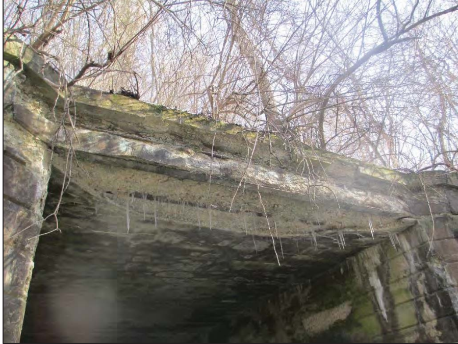
11: General View of the Upstream (West) Fascia
