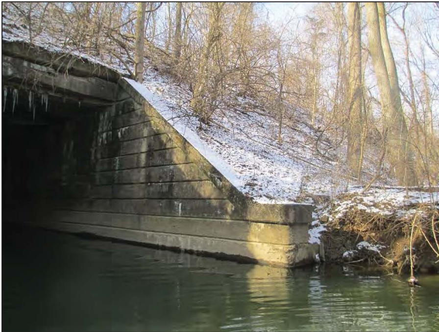
18: General View of the Far Right (Northeast) Wingwall
