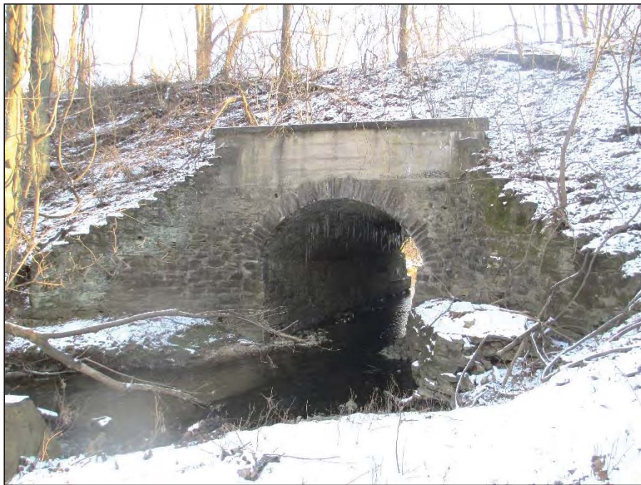
6: Downstream (West) Elevation
