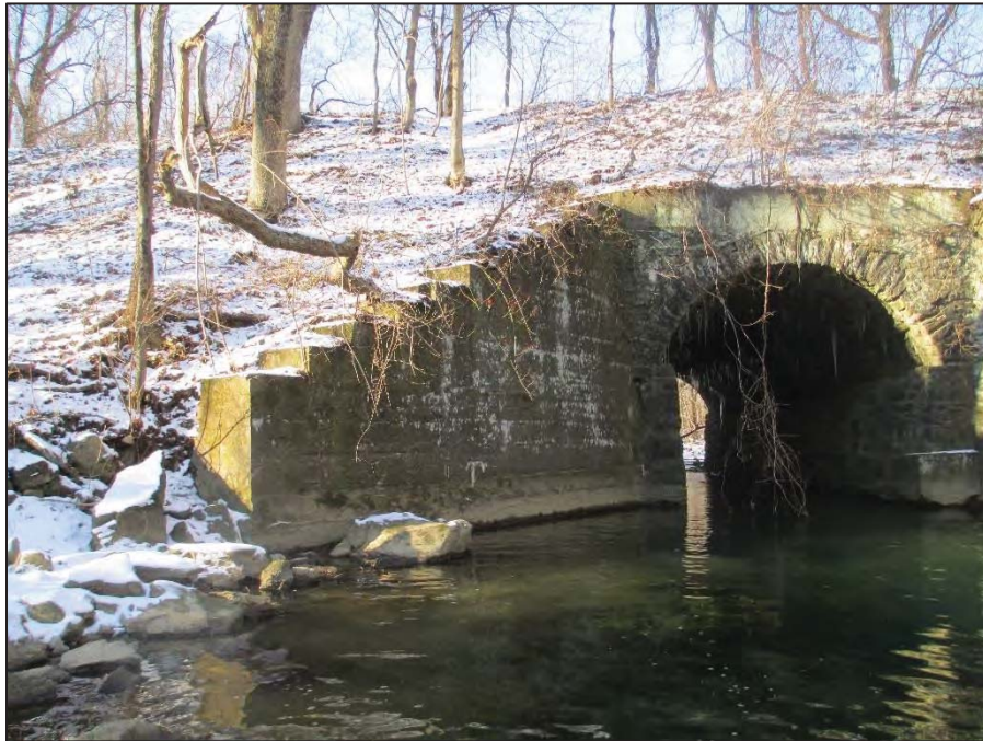
18: General View of the Near Right (Southeast) Wingwall
