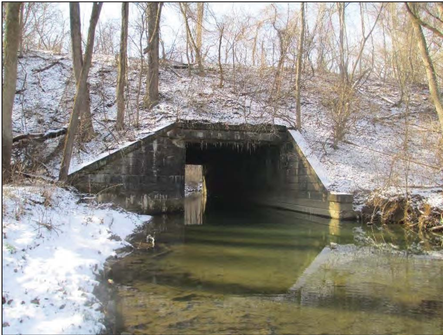
6: Downstream (East) Elevation
