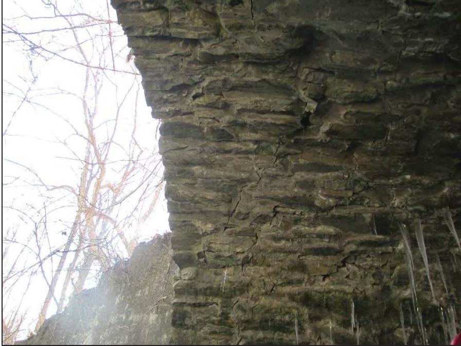
11: General View of the Upstream (East) Arch Ring Underside, Looking Back
