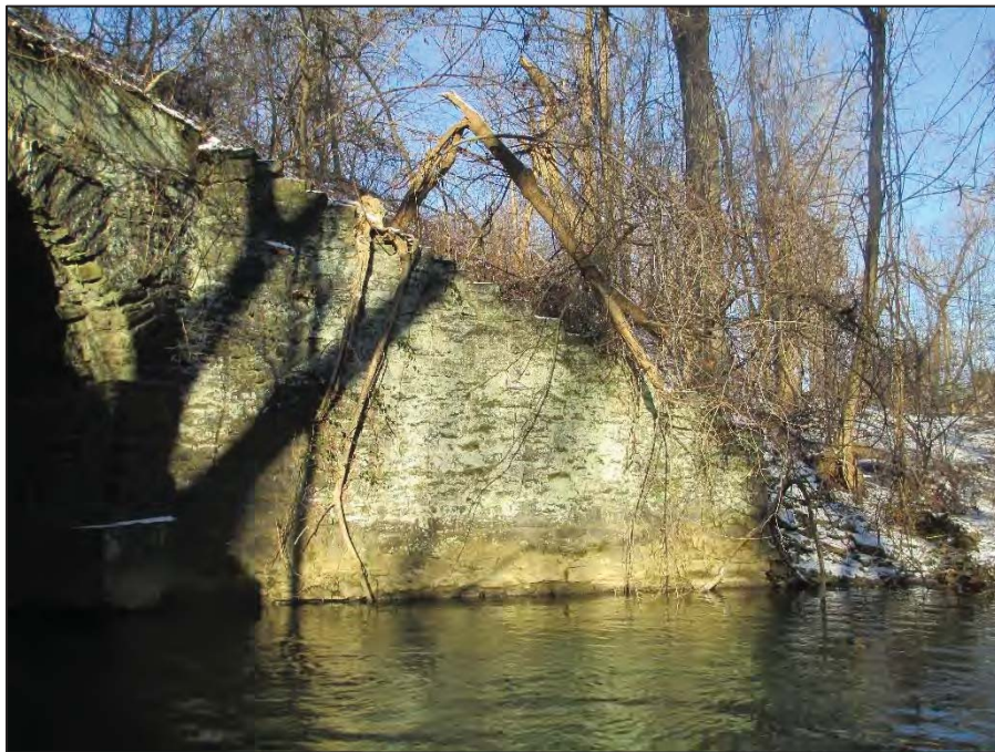
24: General View of the Far Right (Northeast) Wingwall
