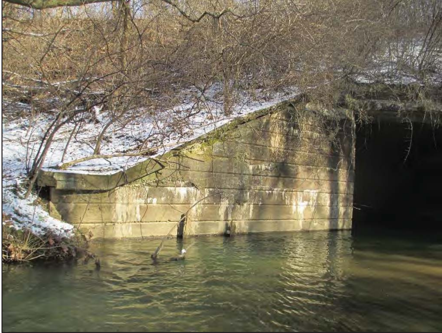
17: General View of the Far Left (Northwest) Wingwall
