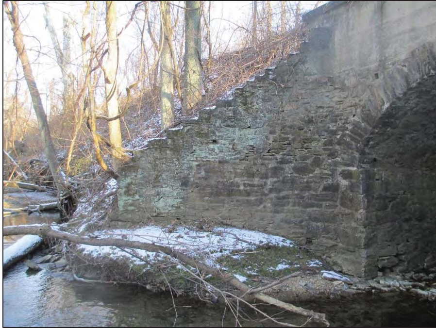
23: General View of the Far Left (Northwest) Wingwall
