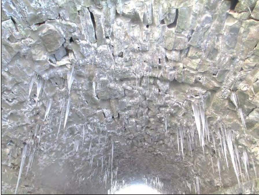
9: General View of the Superstructure Underside, Looking Upstream (East)
