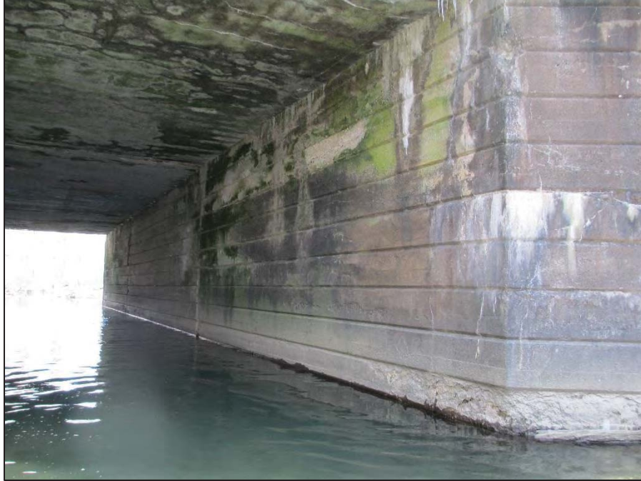
13: General View of the Near (South) Abutment, Looking Downstream
