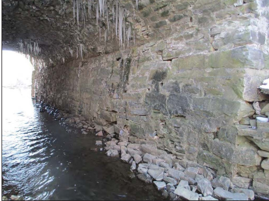
15: General View of the Near (South) Abutment, Looking Upstream
