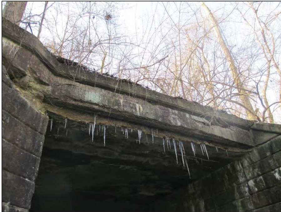
12: General View of the Downstream (East) Fascia
