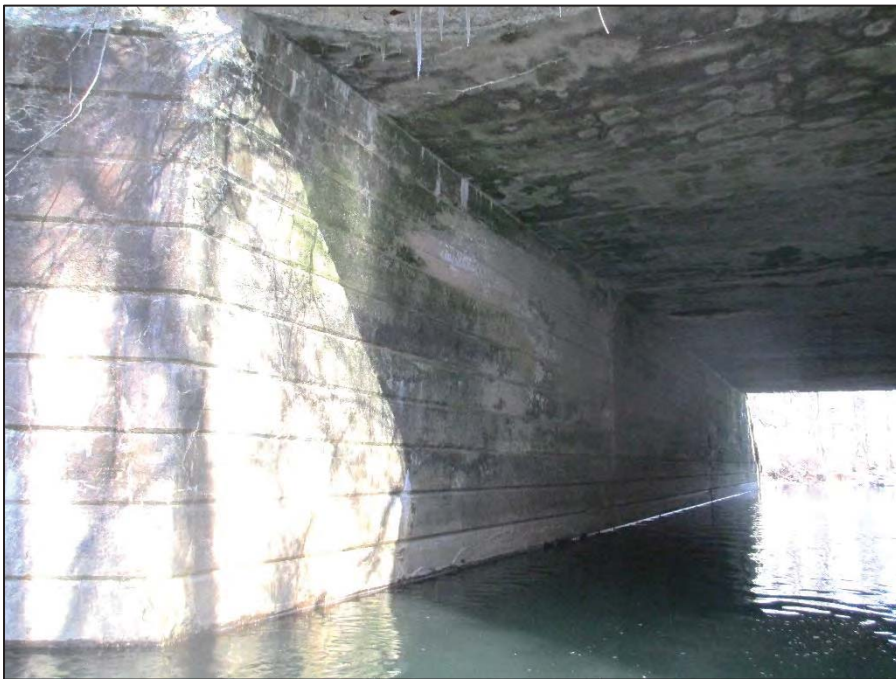
16: General View of the Far (North) Abutment, Looking Downstream
