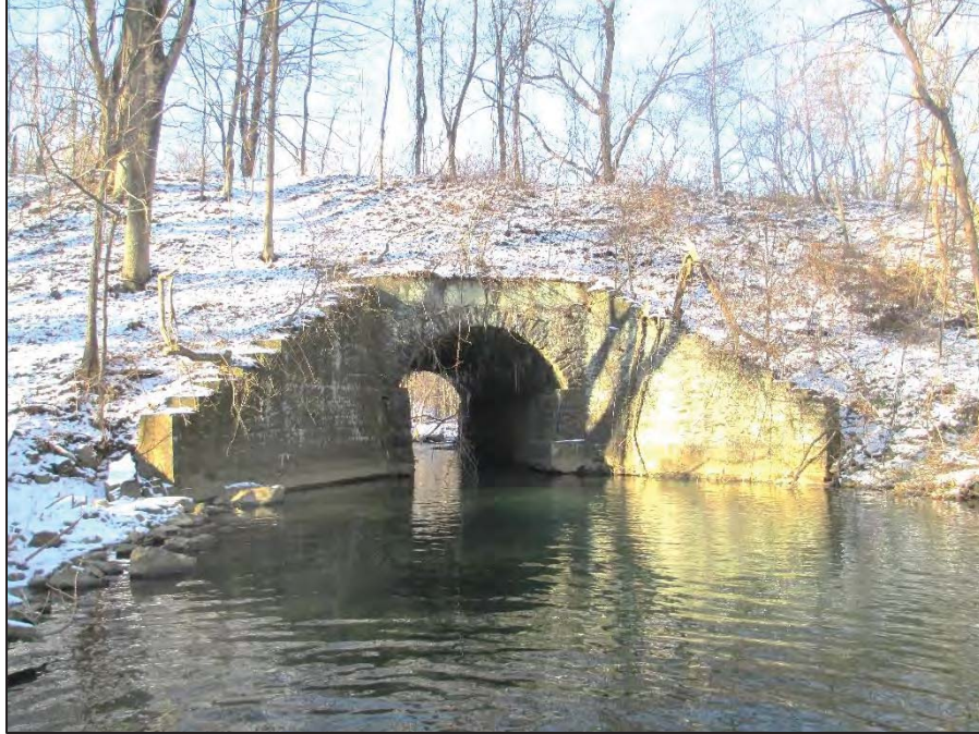
5: Upstream (East) Elevation
