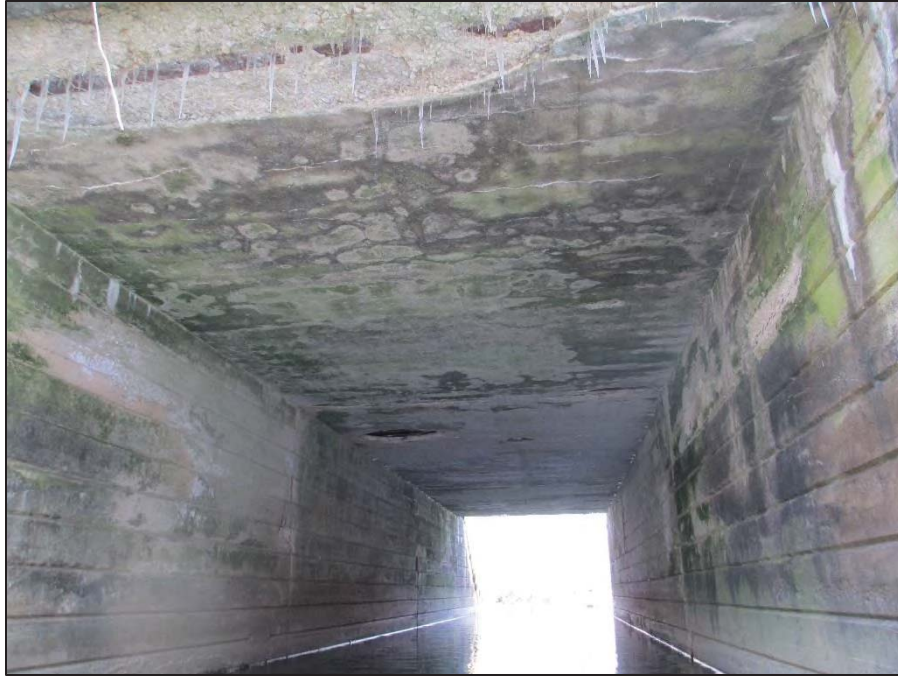
9: General View of the Superstructure Underside, Looking Downstream (East)
