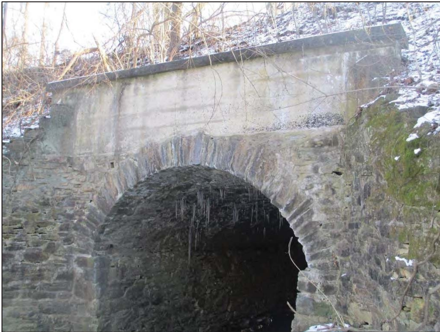
14: General View of the Downstream (West) Spandrel Wall
