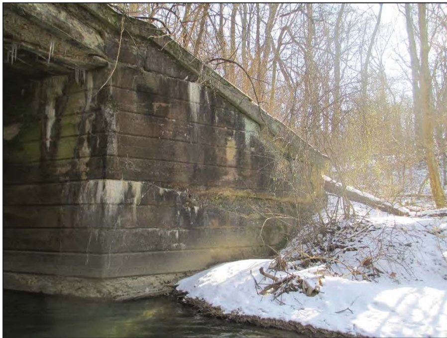
14: General View of the Near Left (Southwest) Wingwall
