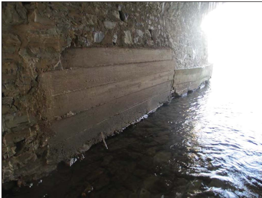
20: General View Far (North) Abutment Apron, Looking Upstream
