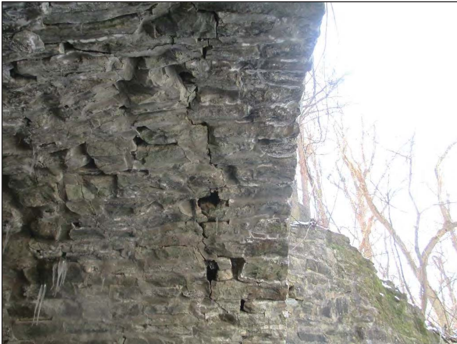
12: General View of the Downstream (West) Arch Ring Underside, Looking Back
