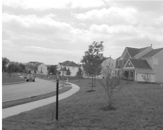
Sidewalks, accompanied by attractive street lighting and trees provide comfortable pedestrian access along Pickering Glen's main entrance road.
