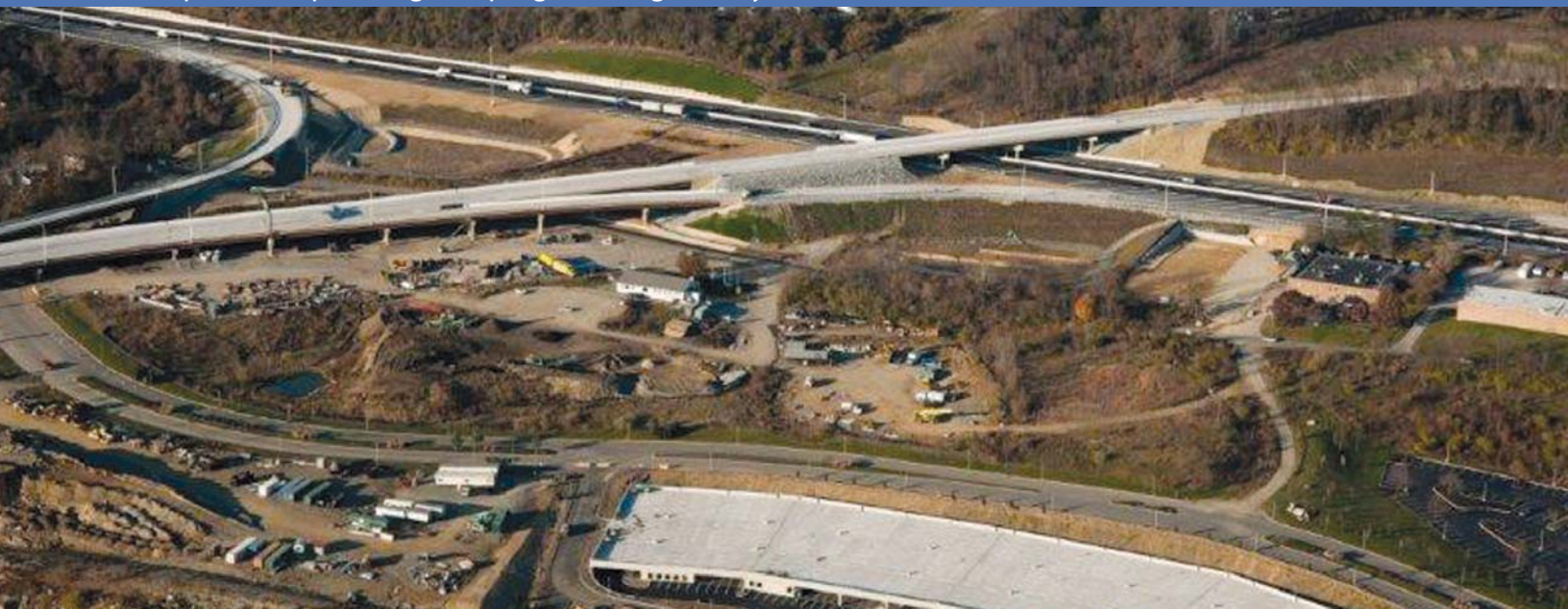
PA Route 29 interchange construction
