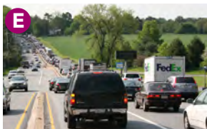
E US 202 Section 100 • PA 926 at US 202 • High Street interchange and Matlack Street intersection improvements
