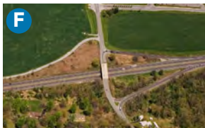
F US 30 Bypass Reconstruction & Widening* Preliminary engineering and final design
