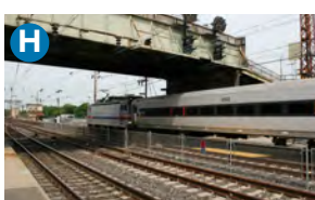
H Darby Road Extension: North Valley Road Bridge* Preliminary engineering and final design
