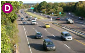
D US 202 Section 200 Operational improvements
