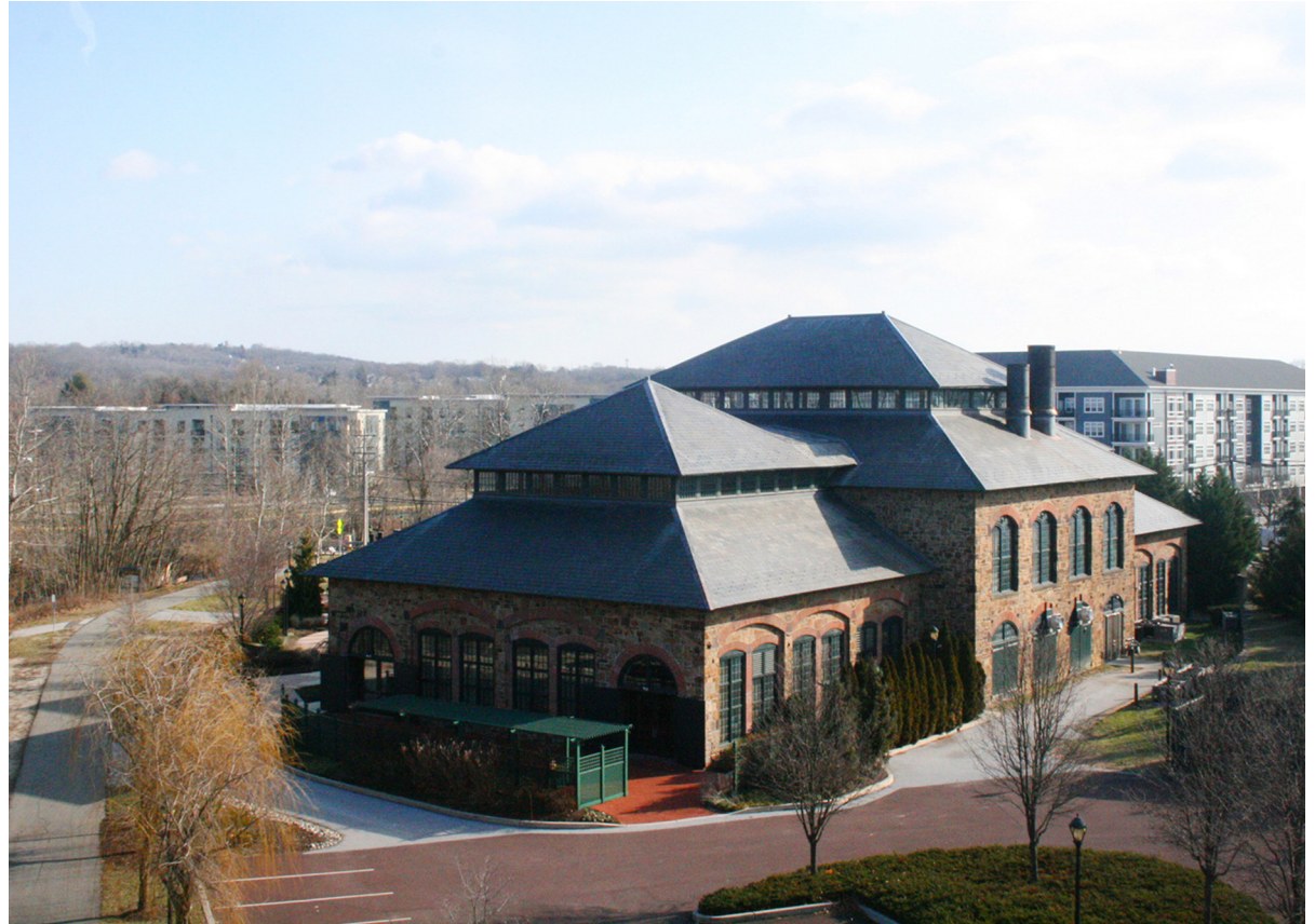
The Foundry in Phoenixville Borough is one of the first and best brownfield revitalization efforts in Chester County and the region.
