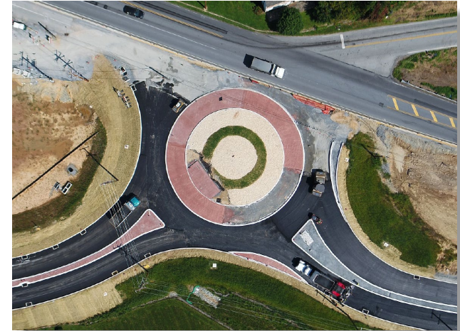
Drone photo of the PA 41 / PA 926 roundabout under construction.
